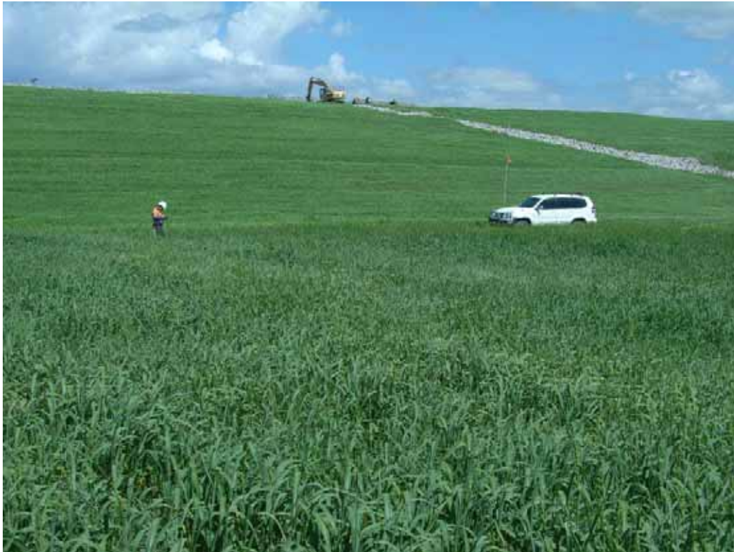
Photograph 2.1 Example of rehabilitation being progressed at HVO South
